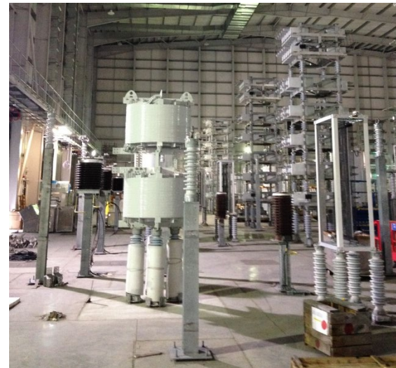
Western Link harmonic filters during construction
