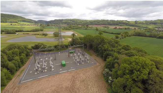
Image : Typical Cable Sealing End Compound (SEC)
