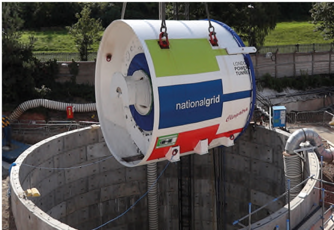
Figure 5.8 Tunnel boring machine being lowered into a vertical shaft
