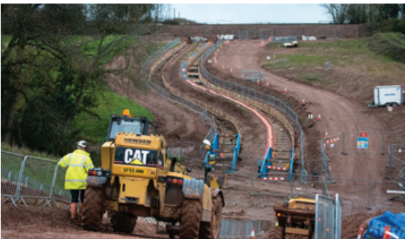
Construction work to replace overhead lines with underground cables
