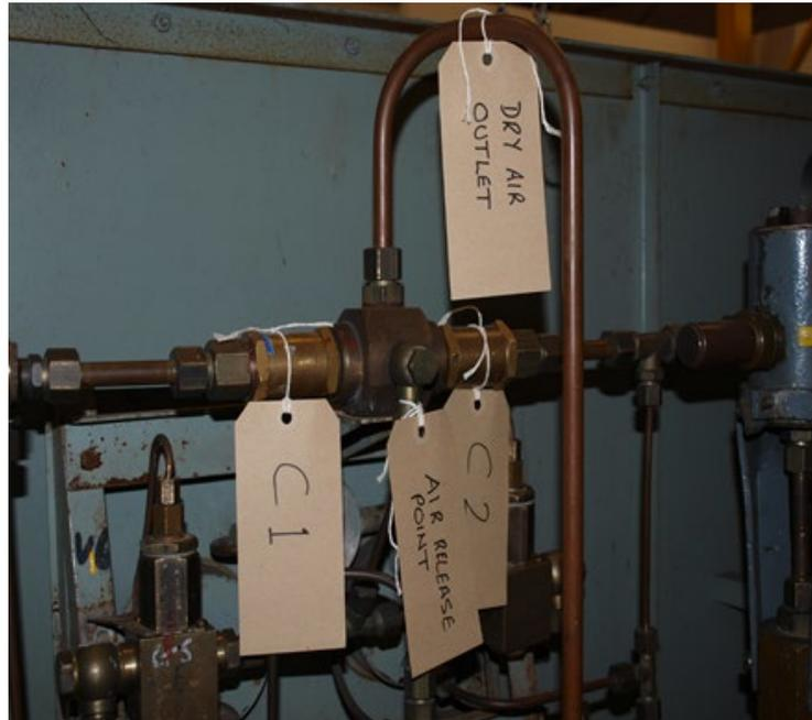
Figure 5.3A – Example of physically identifying the point(s) at which the **Equipment** is to be **Vented** using temporary labels.
