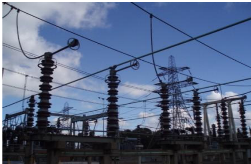
Figure 8.1A – End Rotating Post Busbar Isolators Arranged in Tandem
