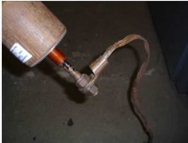
Figure 5.4C – Earth Connection Applied First to Bottom
