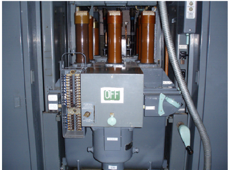
Figure 7.4A - OCB Withdrawn and Umbilical Removed
