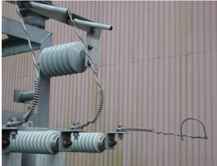
Figure 4.5A - Identifying an Externally Fused Capacitor with a Fuse Operated
