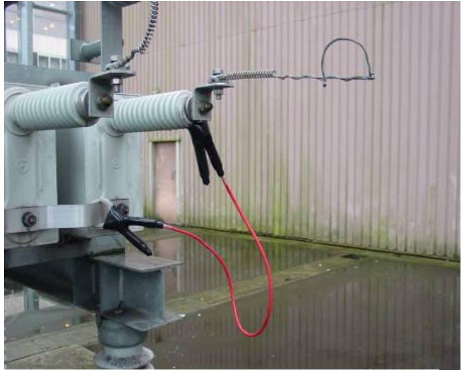
Figure 6.3A – Applying the Clip-on Short Circuiting Lead
