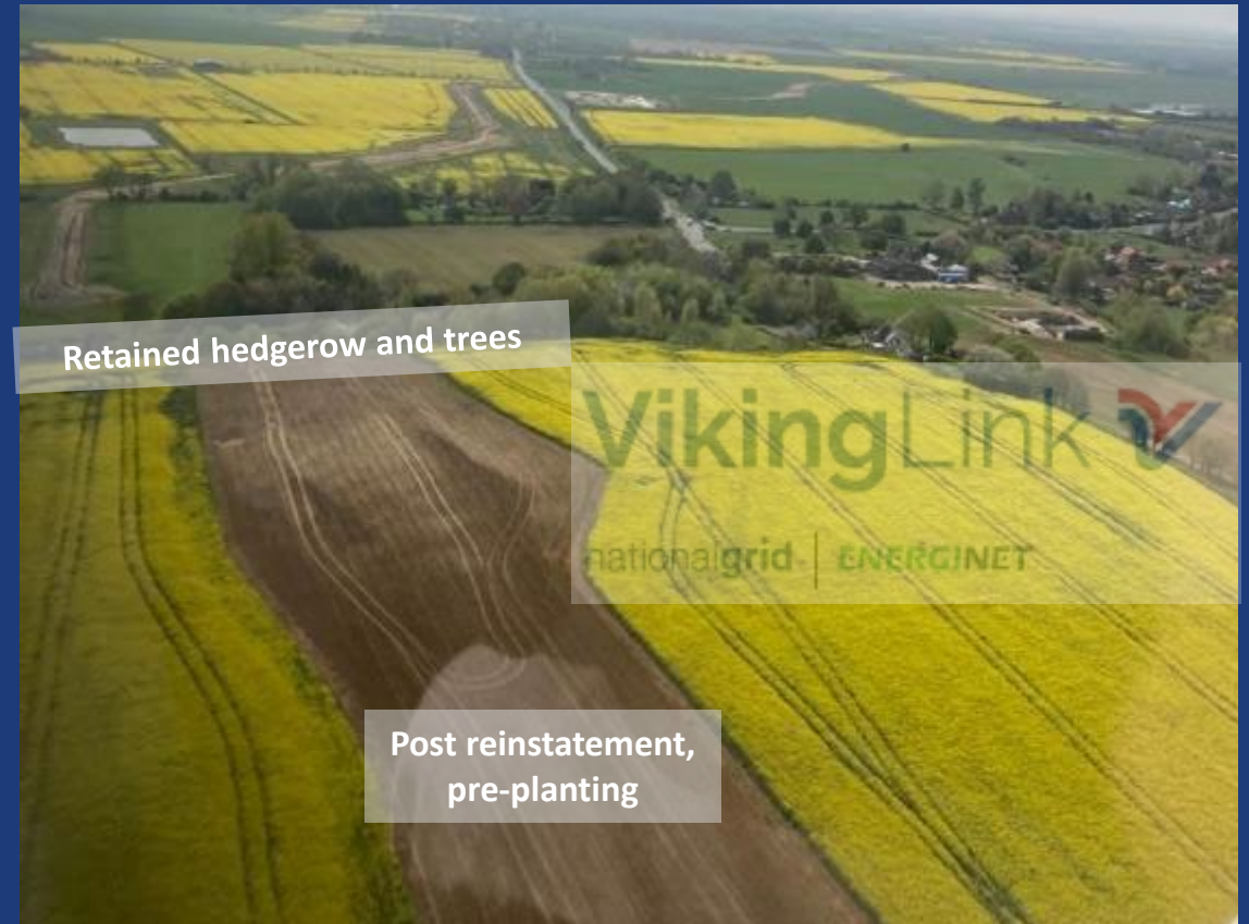
Agricultural land along cable working area reinstated with crops to be seeded by the landowner during the next planting season.
