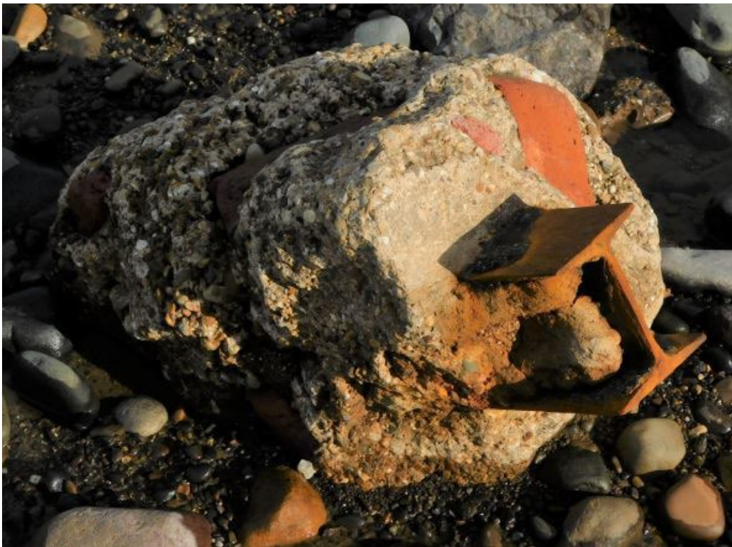
Figure 11 Ex-situ concrete foundation pad with remains of a rolled steel joist (RSJ)
