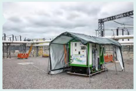
Onsite gas cart used to retro fill existing gas-insulated, high-voltage switchgear, with an alternative low global warming g<sup>2</sup> gas, designed for high-voltage transmission equipment, Richborough Substation, Kent, UK
