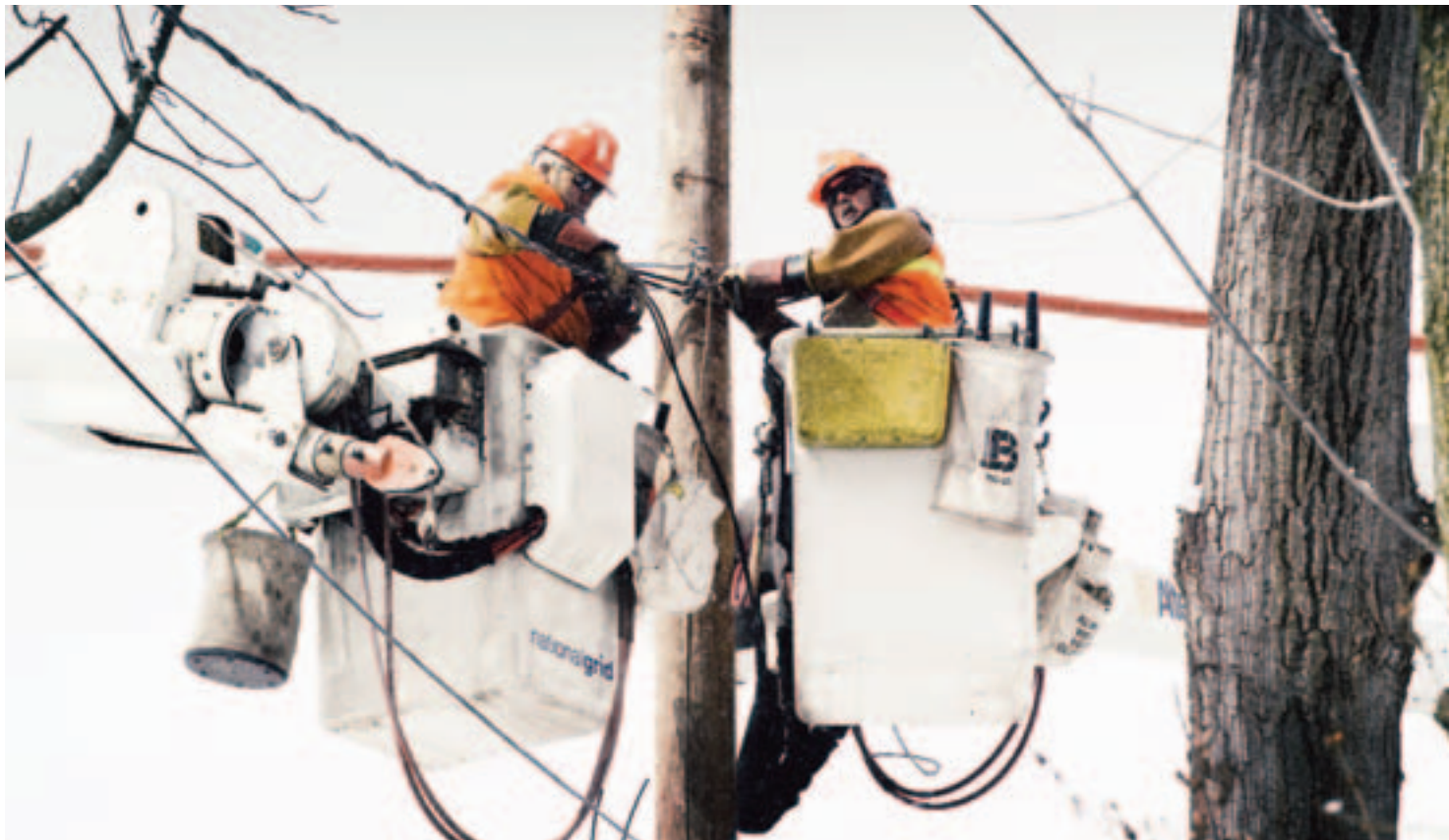
Working on an electricity distribution line.
