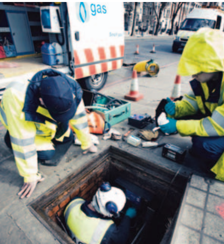
▣ A distribution crew working on an underground governor.
