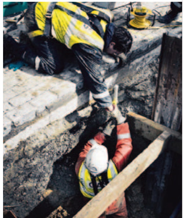
▣ Repairing a gas escape in the highway.
