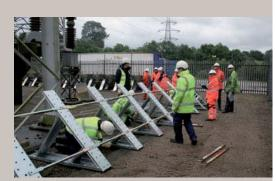
**EMERGENCY:** Temporary flood defences can be deployed at substations
