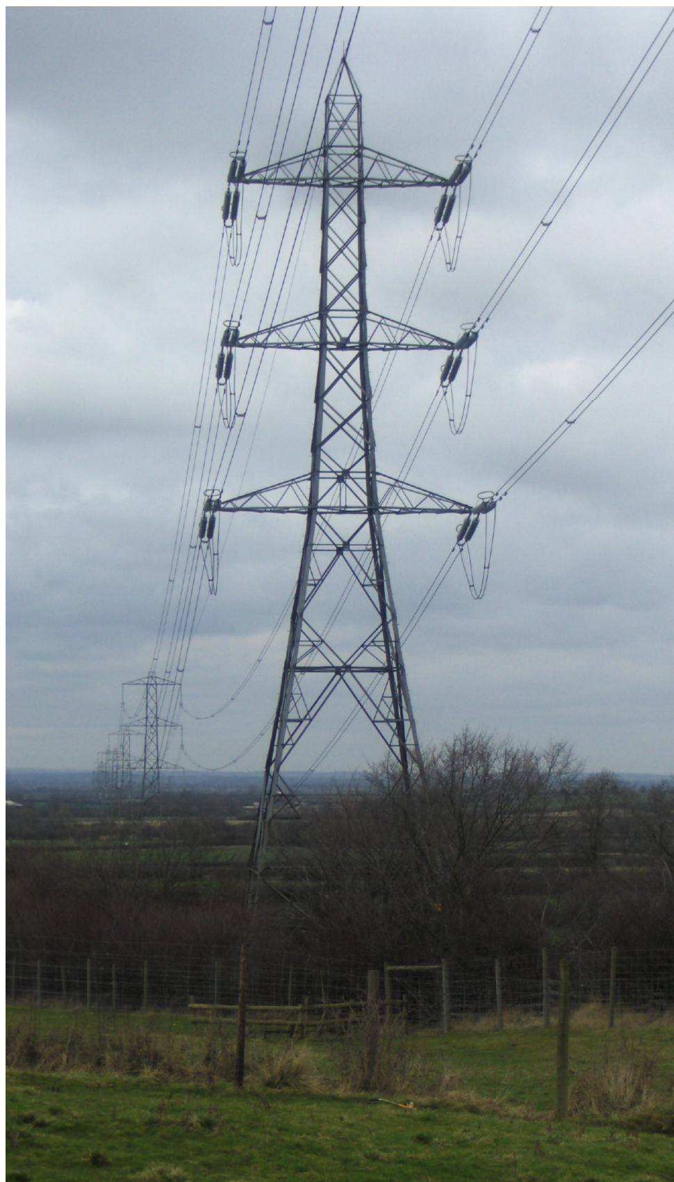
Typical example of an Angle or Deviation Tower
