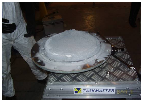
Figure 5.1 A – Example of SF 6 Contamination
