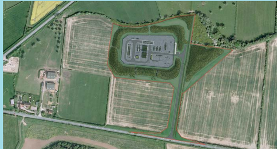
Aerial view of the proposed location of Tirley PRI - original application
