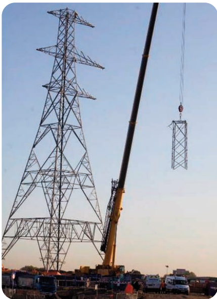
Images from the Olympic Park. From left to right: Tower from overhead line being dismantled, head house during tunnel construction, tunnel prior to cable installation.
